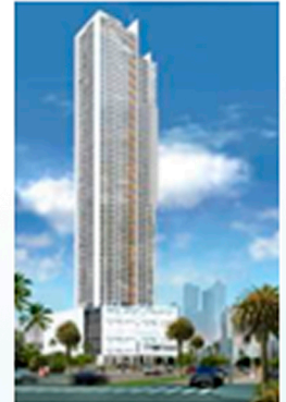
WHITE TOWER $249,900 A $975,000 119 A 390 MTS2 AVE. BALBOA
